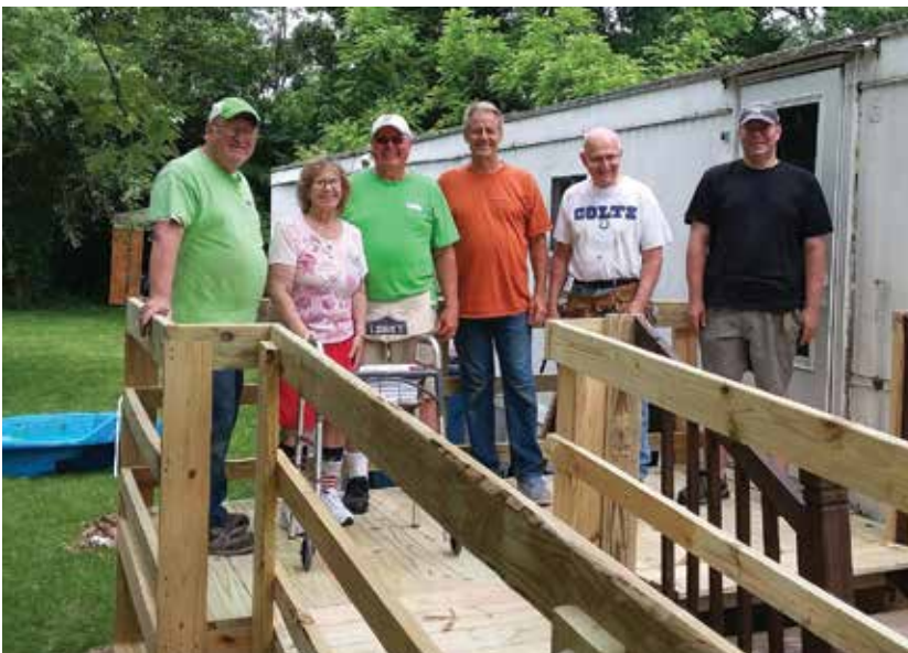
SAWs volunteers smile for the camera with Project Manger John Hunter (far left) after completing a ramp for a deserving recipient.
