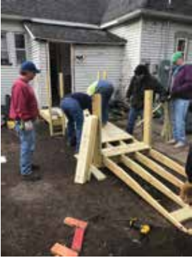
Volunteers in Terre Haute replace an unsafe metal ramp with an ADA-compliant SAWs ramp.
