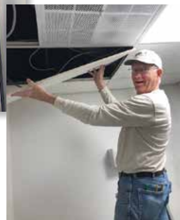
Pete Mohr replaces ceiling tile.
