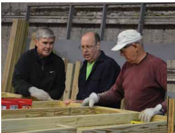
3 Volunteers Greg Morrison, Hal Hefner and Pete Mohr construct a ramp frame.
